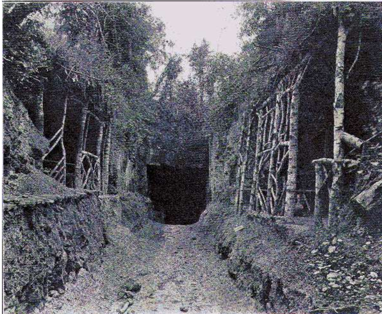
GERMAN DUGOUT ENTRANCE WITH ENTRANCES TO OFFICER'S SHELTERS, HINDENBURG LINE, 1918. THIS SURVIVED THE FINAL ARTILLERY PREPARATION.
